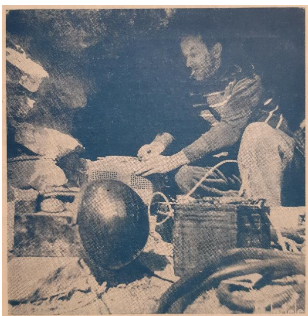
Figure 13: Left: Jean Evenou preparing a recording at the entrance of an abandoned gold mine in Brittany. His tape recorder is a Philips EL 3540. Note the truck battery in the forefront on the right, with the crocodile clips to link the battery to the recorder. Right: Christian Bodin, Georges Lequelllec and Yanette Evenou in the gold mine recording and commenting their expedition. Because the recorder was static at the entrance of the mine, and because the mine was huge, they relied on a telephone line to record their exploration. The telephone is clearly visible, held by Bodin.
